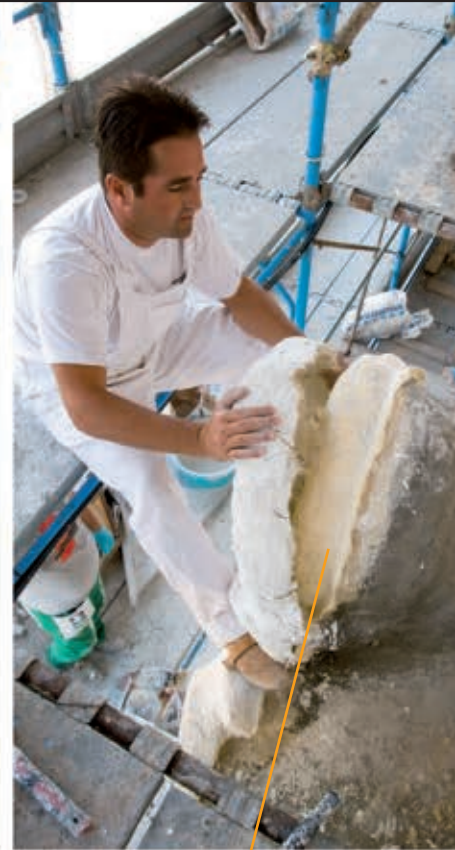
Restaration made with plaster for exterior and with acrylic resins.
